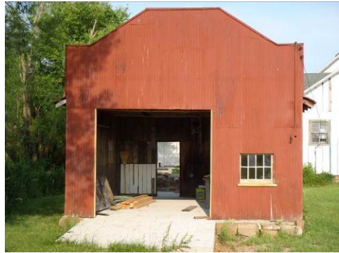
Exterior of Radiator Repair Shop before restoration
