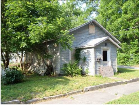
House in Carthage MO that Lowell hopes to make into a train station at Red Oak II
