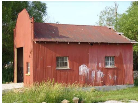
Exterior of Radiator Repair Shop before restoration
