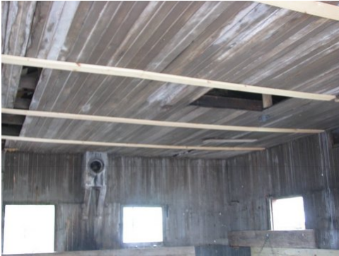
Interior of Radiator Repair Shop before restoration
