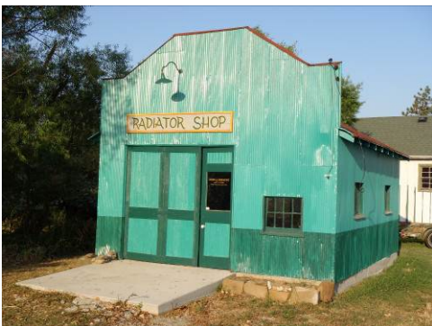
Radiator Shop after painting with front door installed
