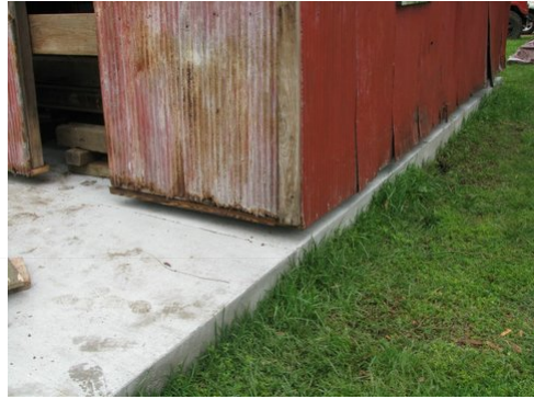
Radiator Shop after lowering onto slab
