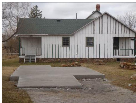
Finished Slab for Radiator Repair Shop
