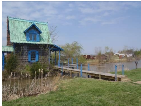
Otis Cabin with New Walking Bridge
