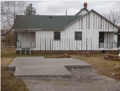
Finished Slab for Radiator Repair Shop
