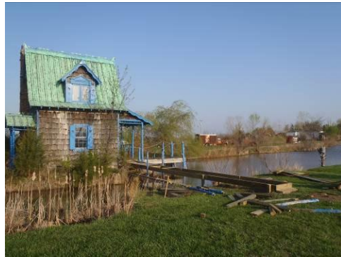
Restoring Walking Bridge to Otis Cabin
