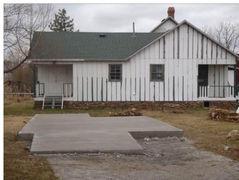
Finished Slab for Radiator Repair Shop
