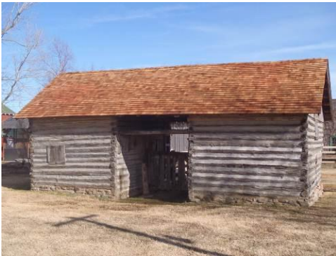
New wood shingle roof on Mule Barn
