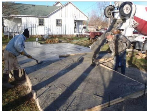
Pouring Slab for Radiator Repair Shop
