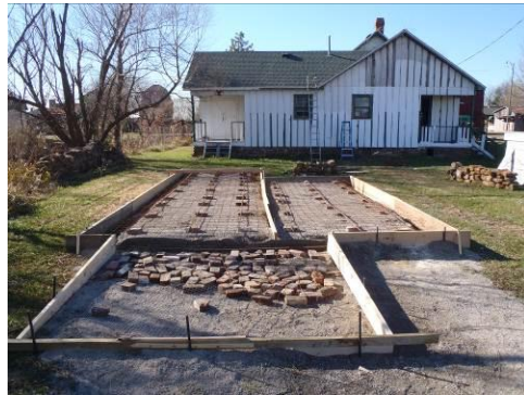
Frame for Slab for Radiator Repair Shop
