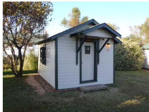
Acorn Unit 1 after renovations
