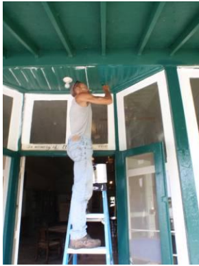
Fresh coat of paint on store front
