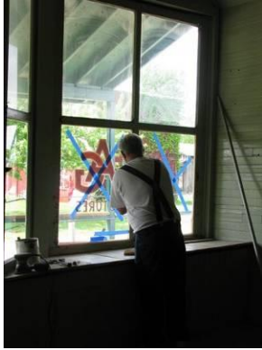
Repairing rotted window frame
