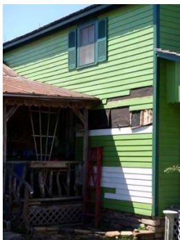
Belle Starr House under renovation
